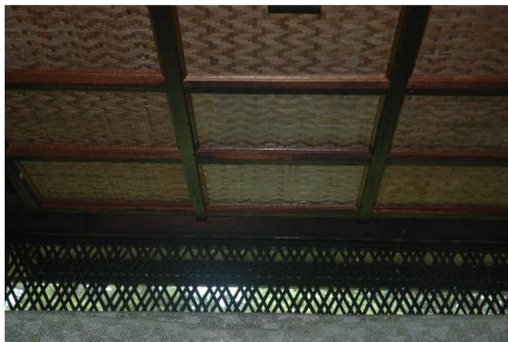
Figure 13: Ventilation openings under roof
