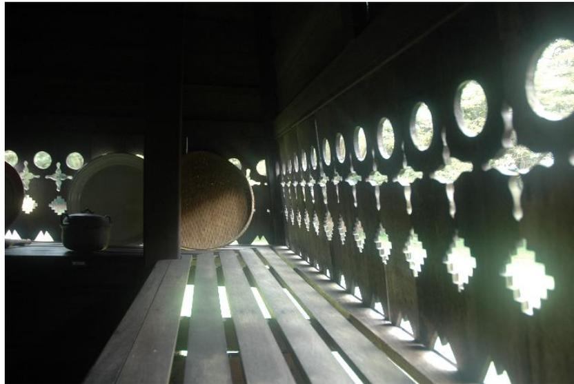
**Figure 15:** Shelves with Ventilation Openings
