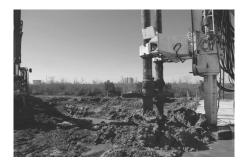
Fig. 20 Deep soil mixing injects cement grout columns deep into poor soil.<u>http://www.defensemedianetwork.com</u>
