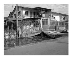
Fig. 16 House settled after a year completion of the construction
