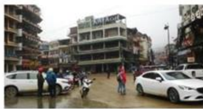
Cluttered and disorderly construction sites on Cau May street
