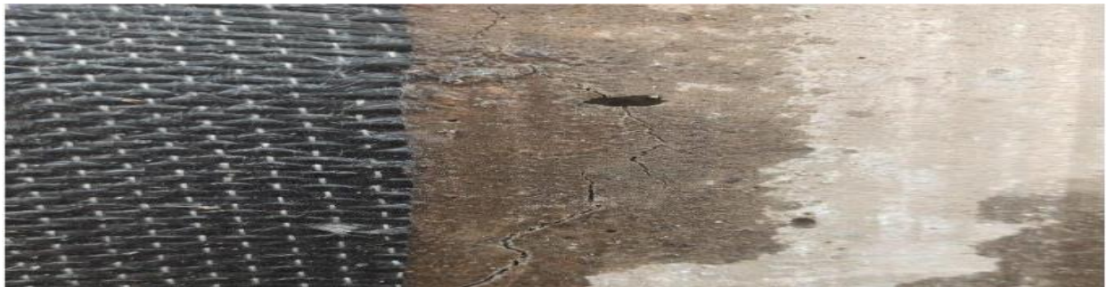
Fig. 4 - First crack on CFRP wrapped beam with 100 mm interval
