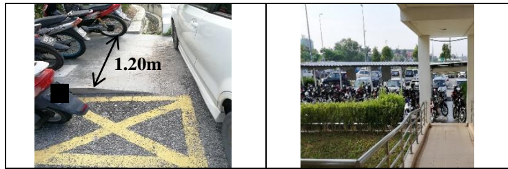
Fig. 4 - The non-compliance on the pedestrian route condition
