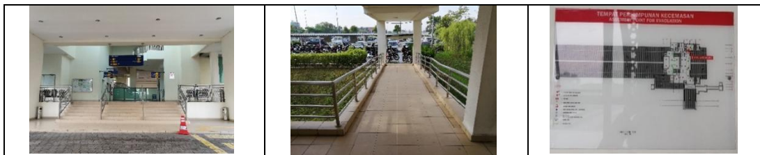
Fig. 5 - The non-compliance on the main entrance and fire safety evacuation procedure
