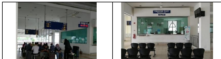
Fig. 6 - The non-compliance on the signages
