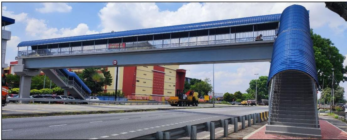
**Fig. 2** UHPFRC pedestrian bridge
