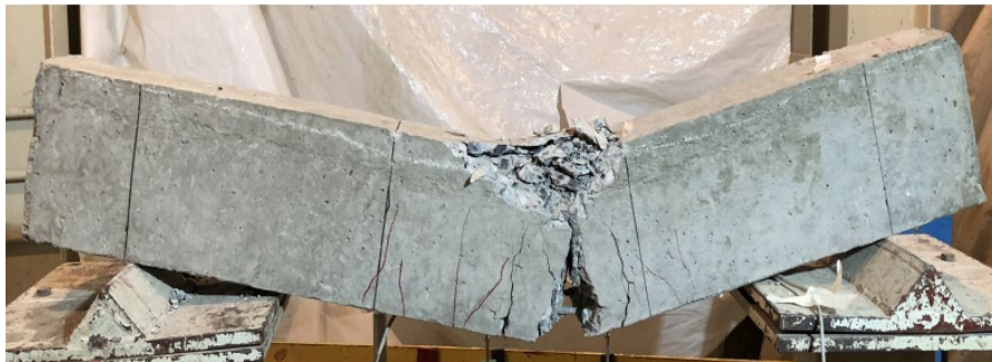
Fig. 9 Failure of ONPRC beam
