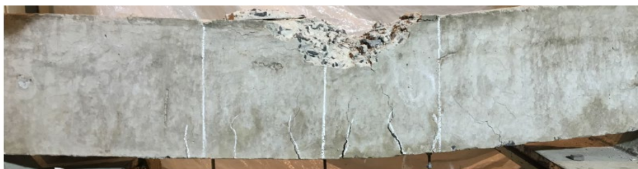
Fig. 18 Crack pattern in AACRPC beam
