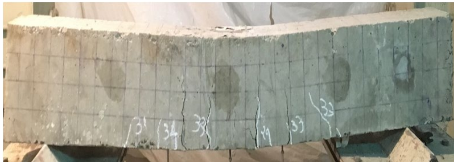
Fig. 12 Crack pattern in GNRPC beam
