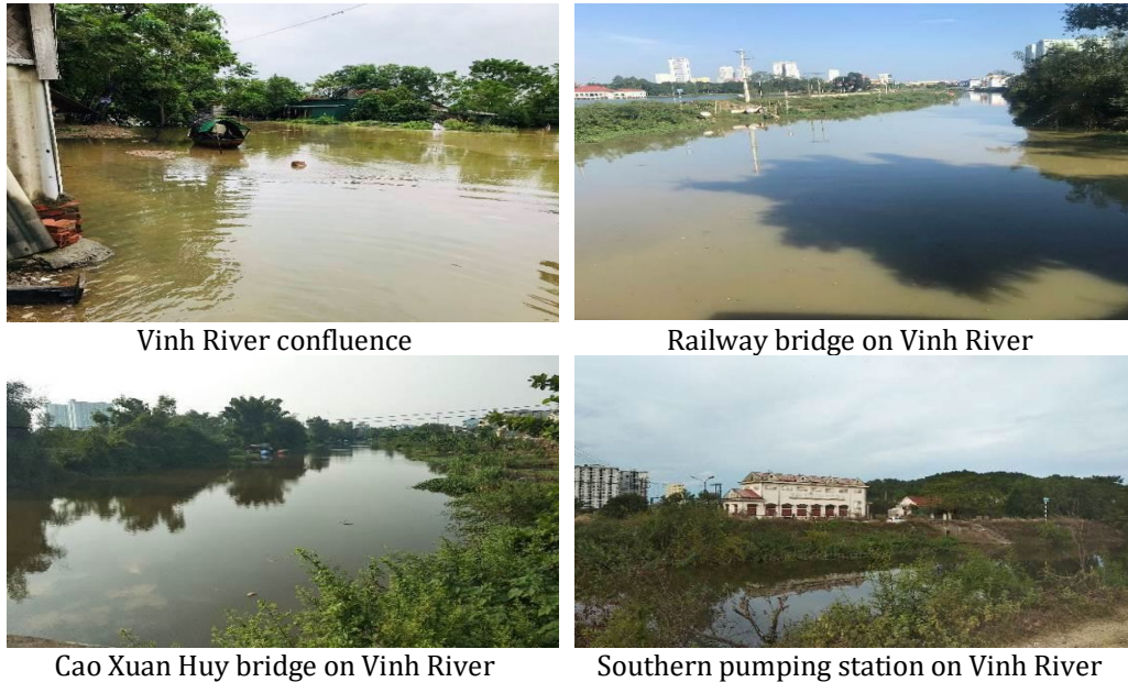
Fig. 3.1 Current status of Vinh river drainage (Source [2,5])
