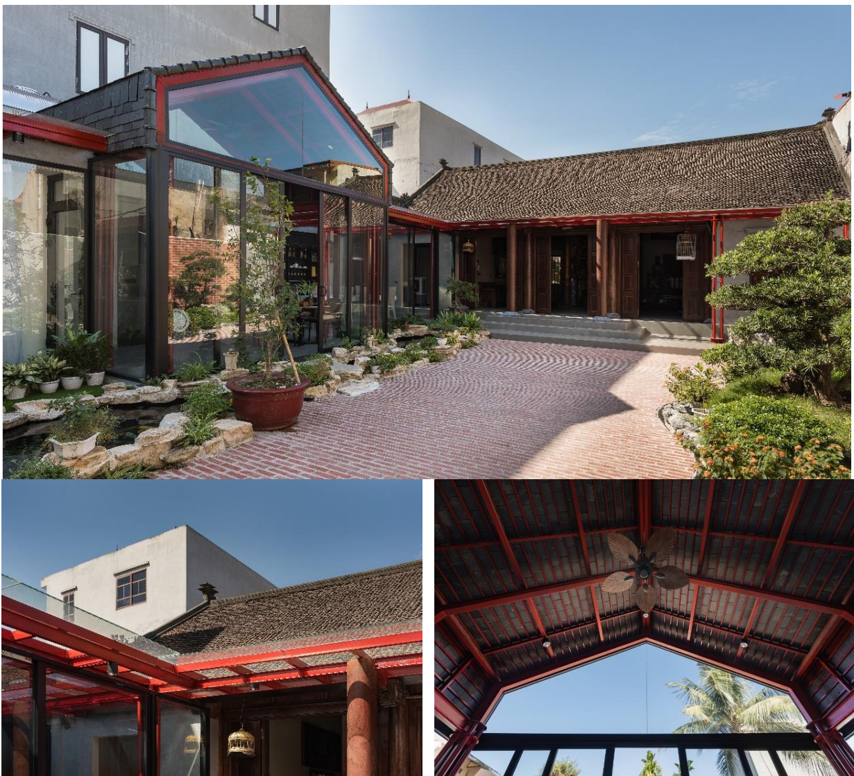
Fig. 12 Some pictures of the project after renovation
