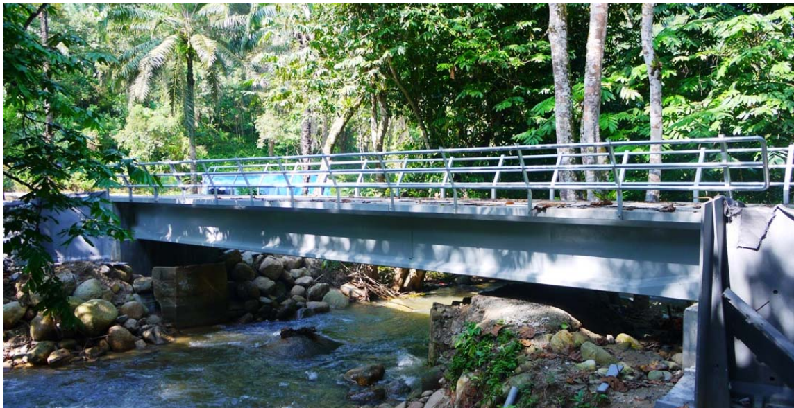
Figure 25: The new UHPFRC bridge at Kampung Ulu Kampar, Gopeng, Perak.
