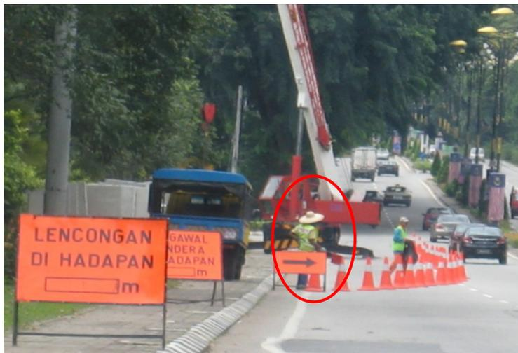
Figure 1. The flagman is placed in the road construction work zone
