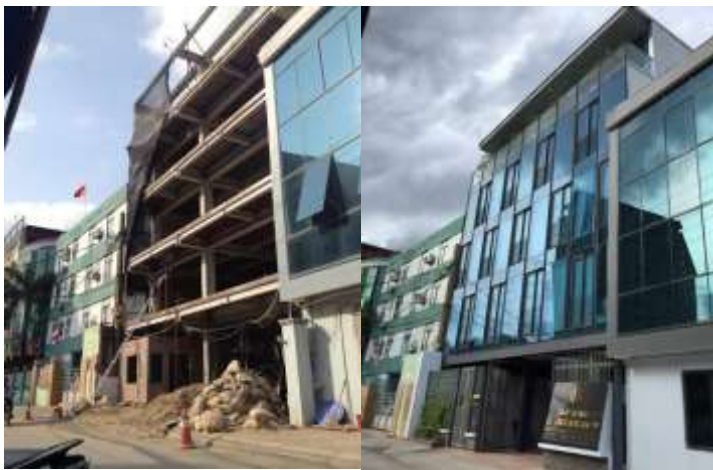
Fig. 15 - (a) During constructing (Company, 2019)
