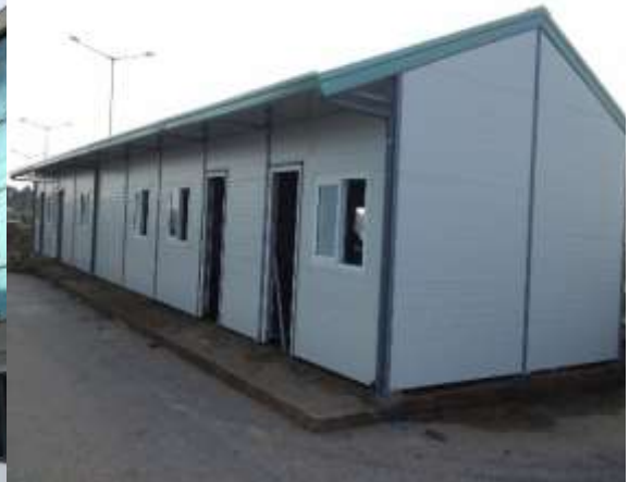
Fig. 17 - Prefab house for workers (company, 2015)
