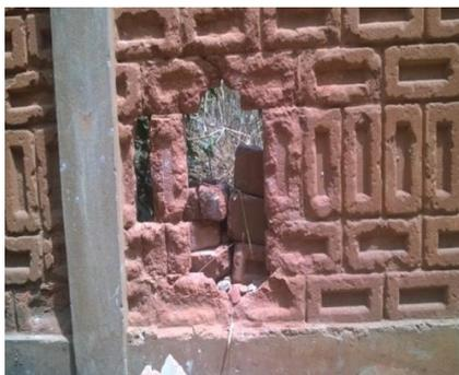
Fig. 3 - Example of wall decrepitude and drilled
