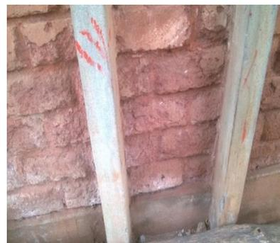
Fig. 4 - Example of crumbling wall
