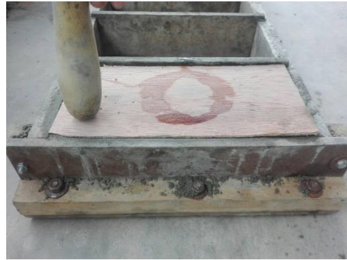
Fig. 5 Flattening the surface of the brick with a plywood to prevent uneven surface.
