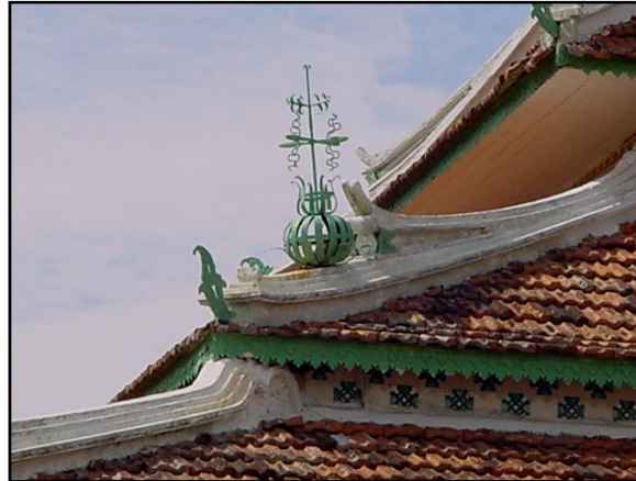
Figure 4. Lower and upper attached roof overhangs.
