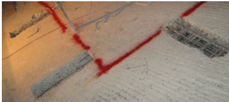
Fig. 4 - Cutting zone and locking pockets area
