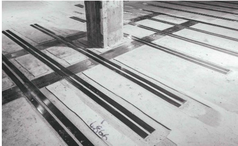
Fig. 7 - Slab strengthening with fiber-reinforced polymer [28]
