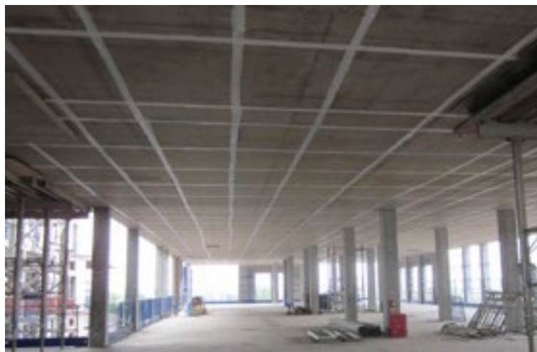
Fig. 3 - The marking of tendon locations [24]
