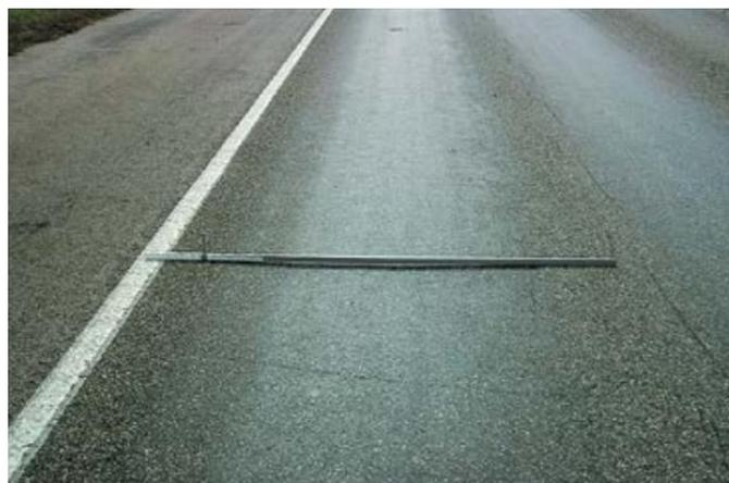
**Fig. 3 - Rutting or permanent deformation in flexible pavement [13]**
