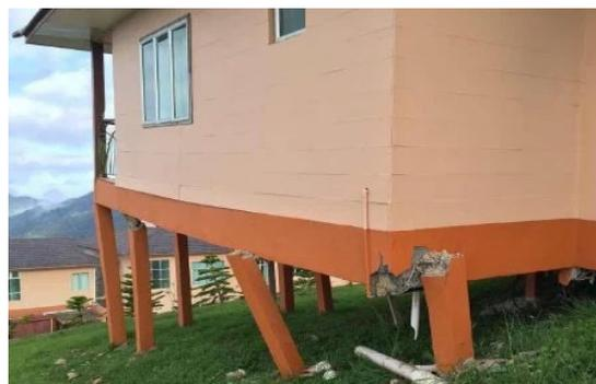
**Fig. 2 - Stilt house damaged due to short column effect**
