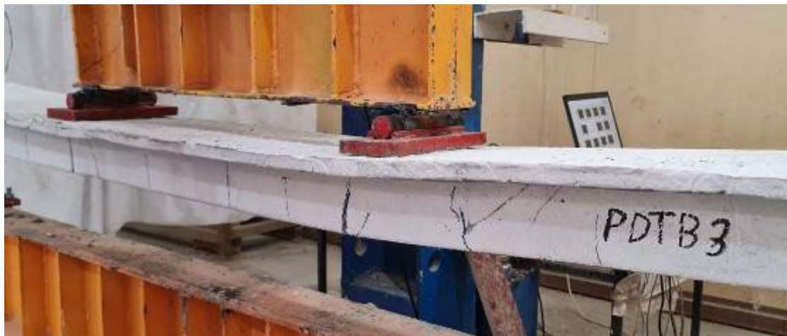
Fig. 18 Places of appearance of crack causing failure (from experimental)
