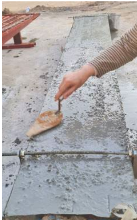
Fig. 3 Casting of mold
