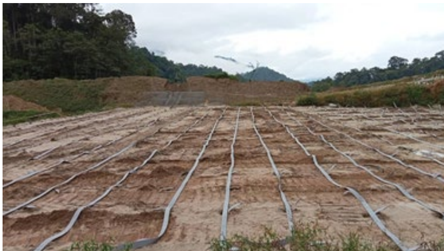
Fig. 7 Horizontal drains setting out
