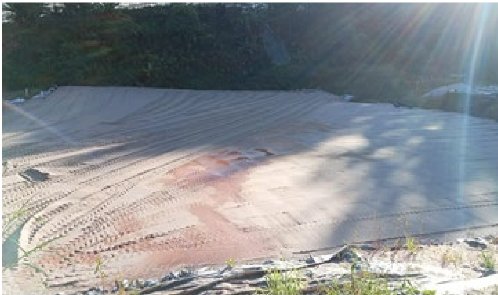
Fig. 3 Project site after site preparation
