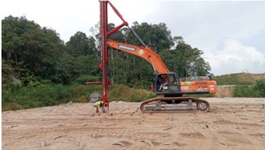
Fig. 6 Installation of vertical drains
