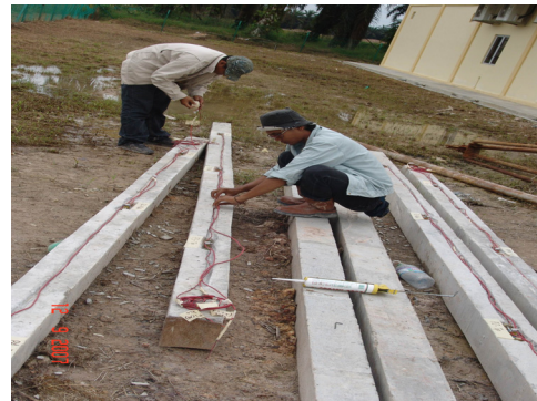
Fig. 2: Installing the strain gauge prior to driving
