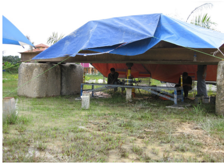
Fig. 3: S-M pile loading test is underway
