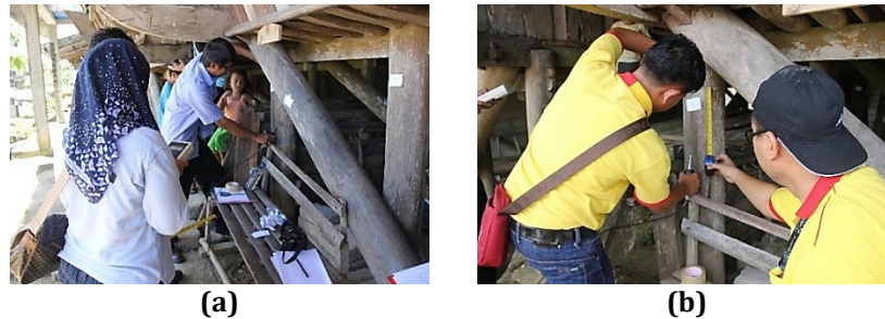
Fig. 5 The process of collecting velocity data on existing buildings with non-destructive testing methods (a) Botohilitano existing building; (b) Bawomataluo existing building
