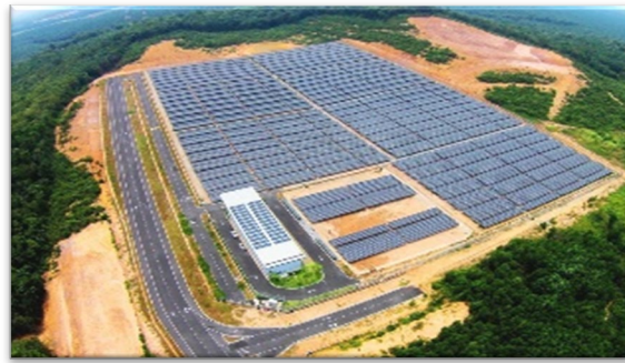
Fig. 1 8 MWp Gading Kencana Ayer Keroh solar farm overview [12]
