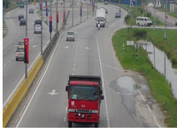
Fig. 1 Site A: Federal Road FT050 KM15
