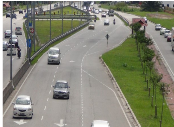
Fig. 2 Site B: Federal Road FT050 KM16.
