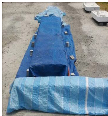
Fig. 6 - Curing of the beam after casting.
