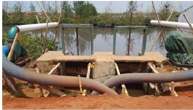
Fig. 11 - The current pump house
