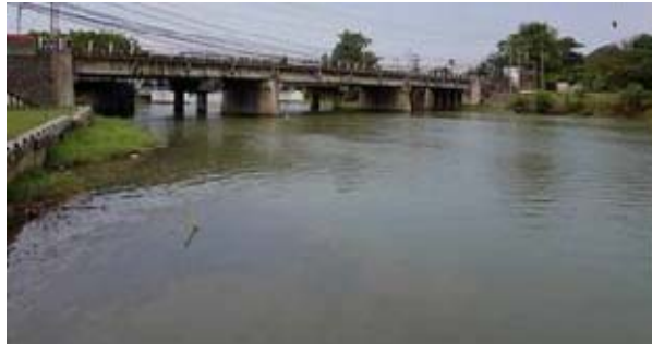
Fig. 5 - Sengkarang river is a completely different river than Meduri river
