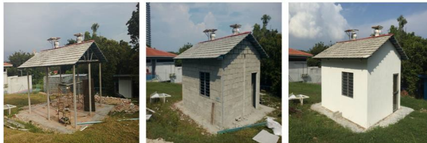
Fig. 4 - Construction of the real scale model for the empirical study
