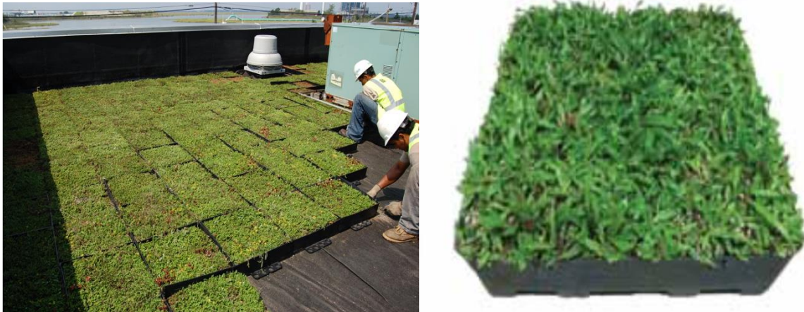
Fig. 3 - Examples of modular extensive green roof
