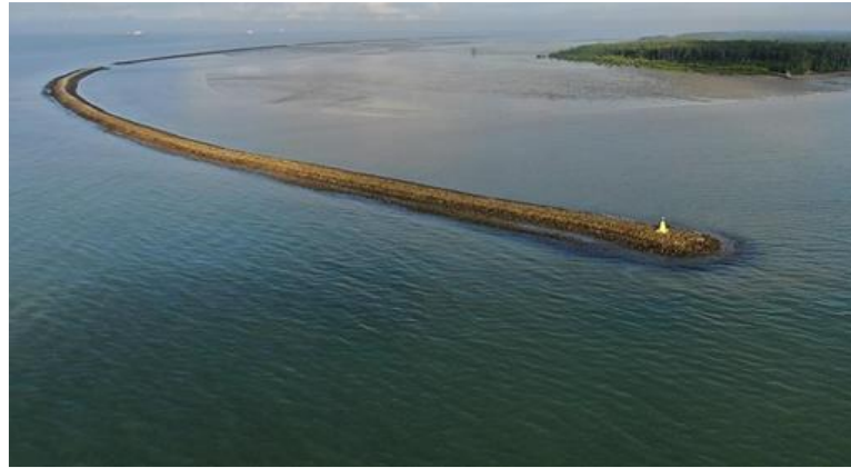
Fig. 13 - Offshore breakwaters constructed at Tanjung Piai, Johor
