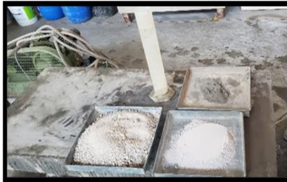
Fig. 3 - Materials preparation used for mixing of CLSM
