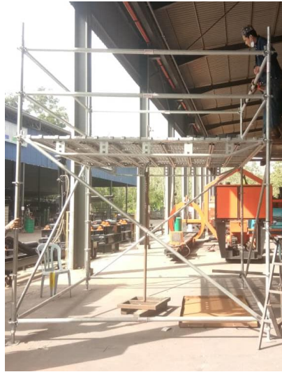
Fig. 2 - Single bay - one story of ARMS Scaffold built
