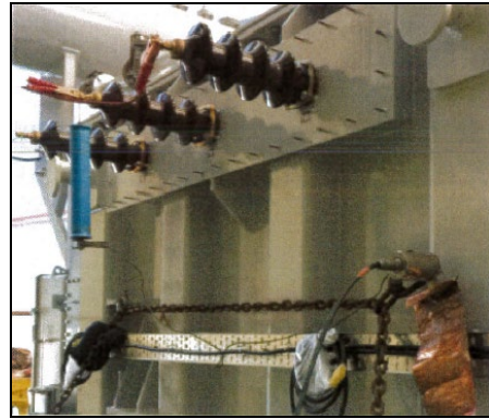
Fig. 2.5 - Installation of shunt for current measurement
