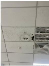
The defect that has occurred at level 1 south east tower building are dampness
