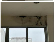
The defect that has occurred at level 1 south east tower building are algae growth and dampness
