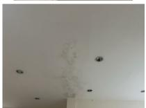
The defect that has occurred at level 1 south east tower building is dampness.
