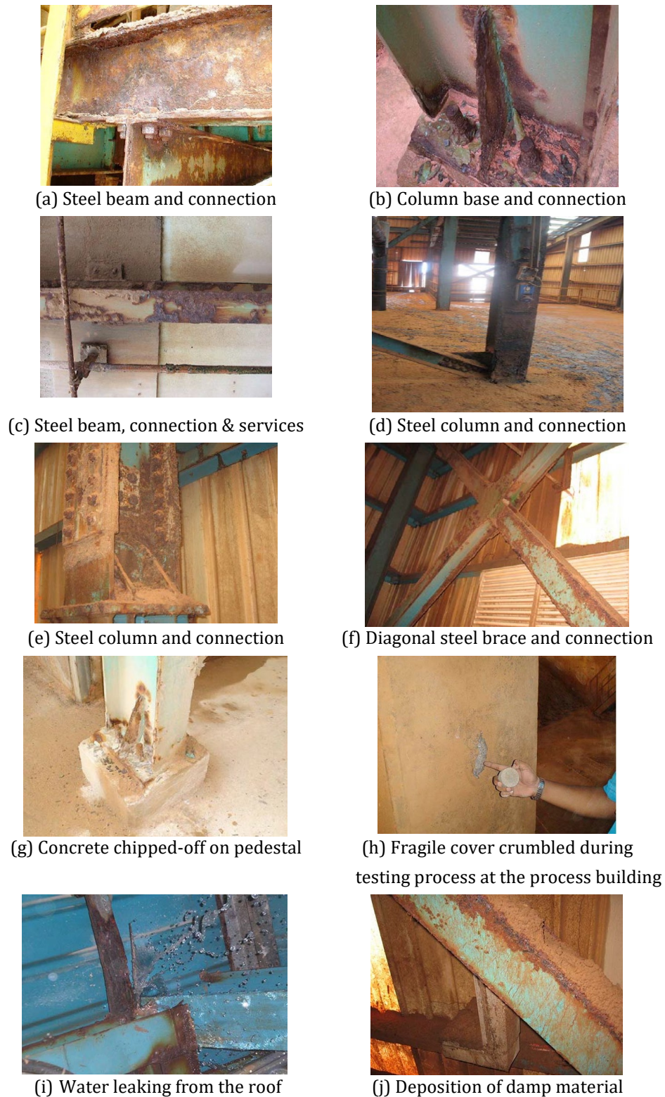
Fig. 2 Observation on structure defects
