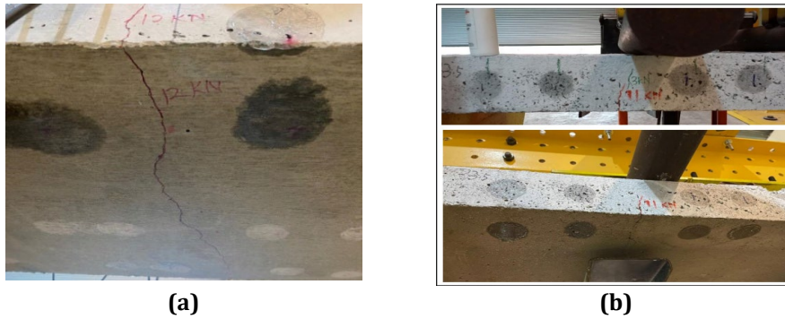
Fig. 5 Crack mapping (a) slab 1; (b) slab 2
