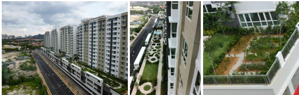
Figure 2 : Rooftop garden at case study building (Maryanti, 2013).
