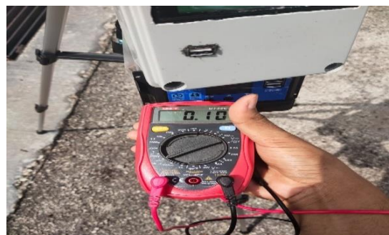
Figure 8: Current Reading for Solar Panel
