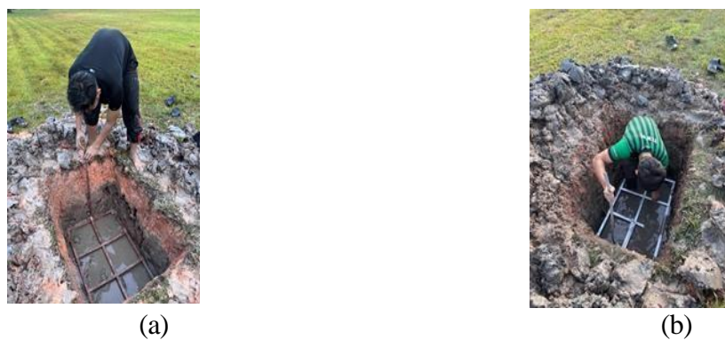
Fig. 4 Grid installation (a) Copper grid grounding, (b) Aluminium grid grounding
