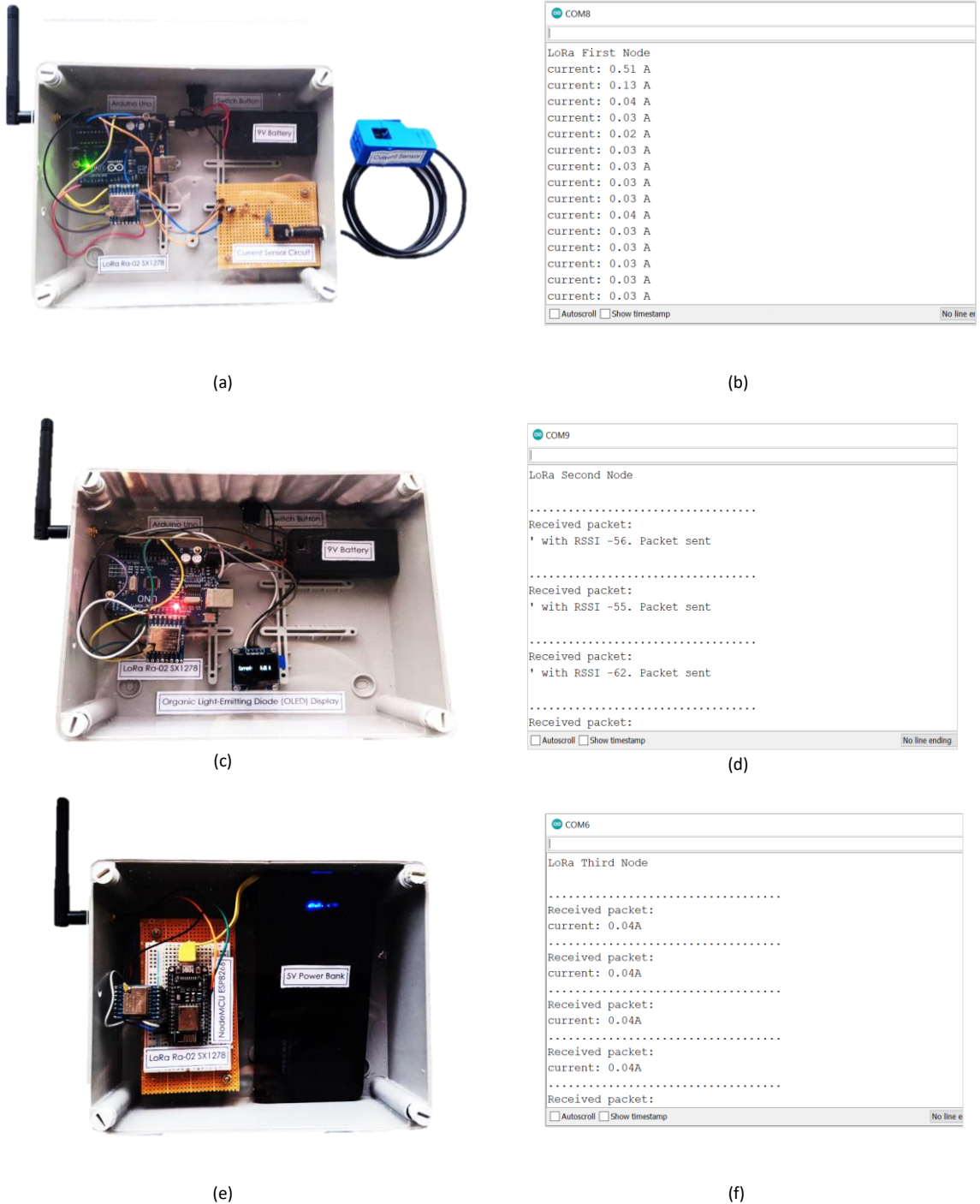
Figure 2: Connection between sensor nodes and gateway (a) First node (transmitter) hardware setup (b) First node serial monitor displays of current sensor readings (c) Second node (mediator) hardware setup (d) Second node serial monitor display of data received and transmitted (e) Gateway (receiver) hardware setup (f) Gateway serial monitor display of current data received
