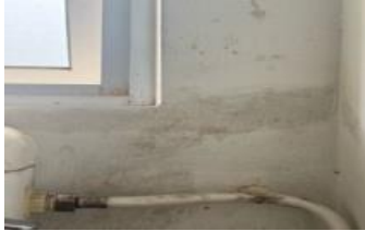
Water leakage
