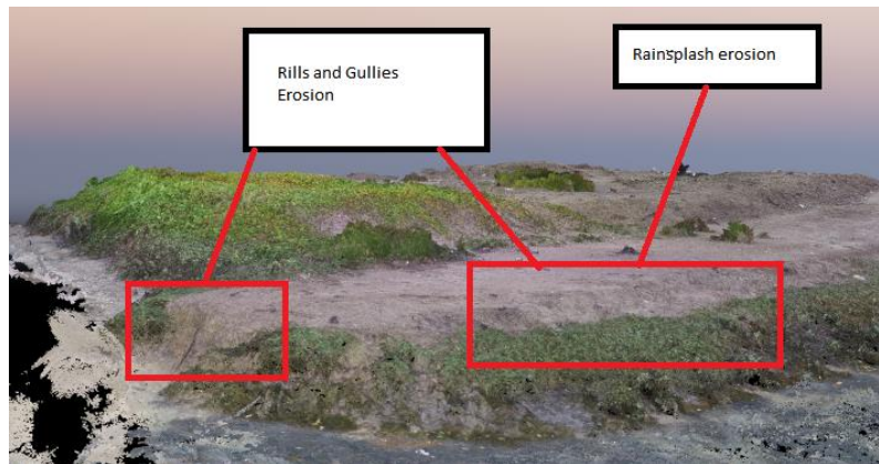
Figure 15: Location of the erosion occurred
