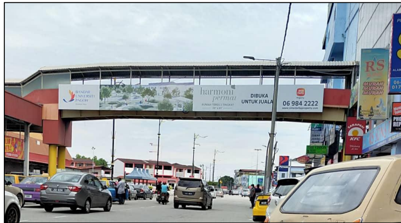
Figure 3: Footbridge in front of the Astaka Shopping Mall, Muar
