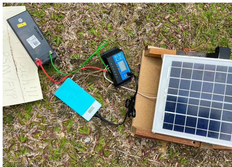
Figure 5: Charging load testing.
