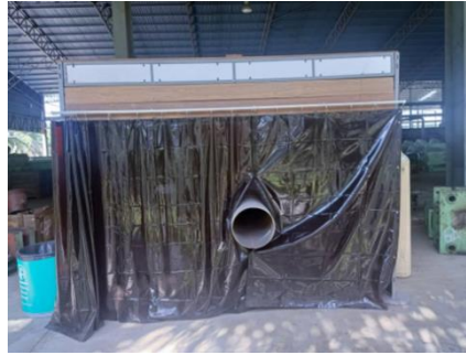
Figure 6: The Installation of Welding Strip Curtain
