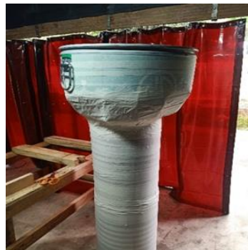
Figure 4: The Installation of the Funnel
