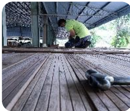
Figure 2: Installation of Wooden Board as a Roof of Soundproof Room
