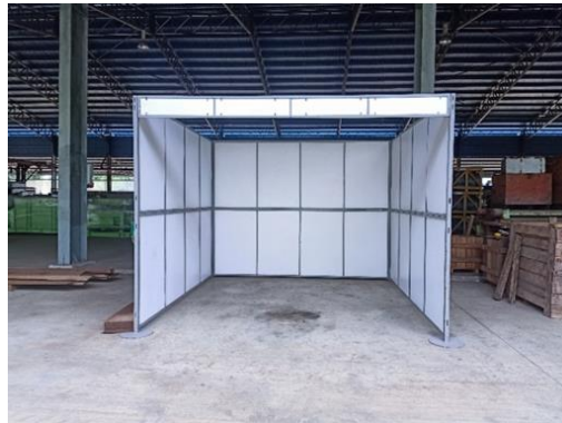
Figure 1: Installation of the Exhibition Partition Booth Part
