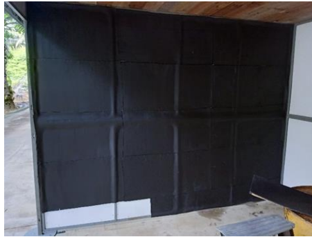
Figure 3: The Installation Process of Acoustic
