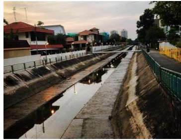
Figure 2 : Linkwise Technology provide a flood monitoring system in Singapore [15]
