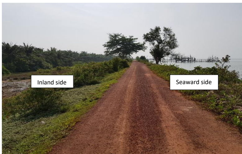
Figure 1: Embankment at Senggarang, Batu Pahat
