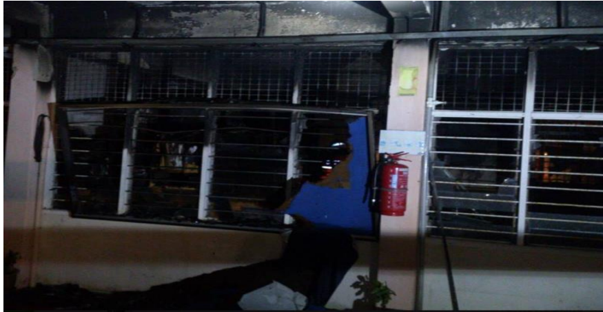
Fig.1 The position of fire extinguisher
