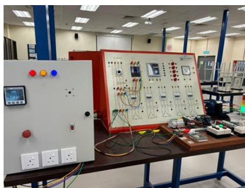
Fig. 4 Testing with Power Factor Correction Trainer
