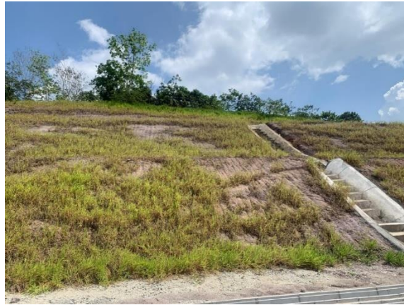
Fig. 1 Hydroseeding Slope Protection
