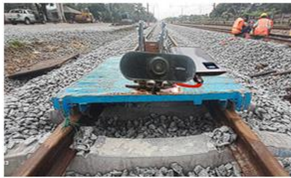
(a) Final Project in Construction Railway
